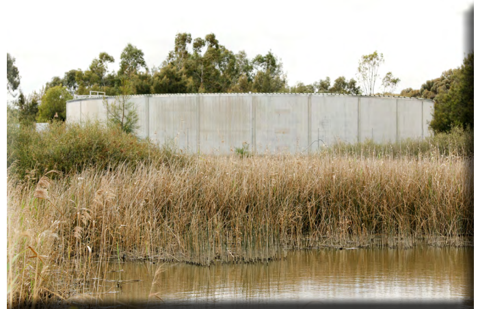
Mawson Lakes water tank
