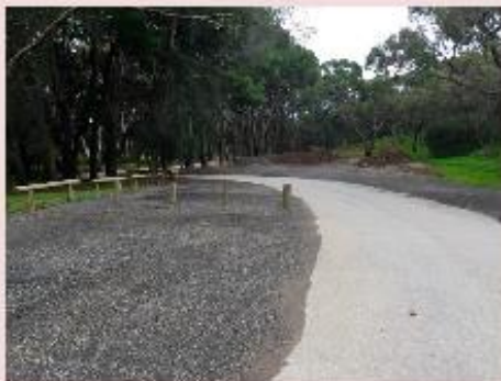
Harry Bowey, Salisbury Park Car Park Renewal, recycling road pavement
