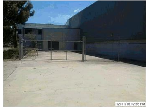
Generator Room – External View
