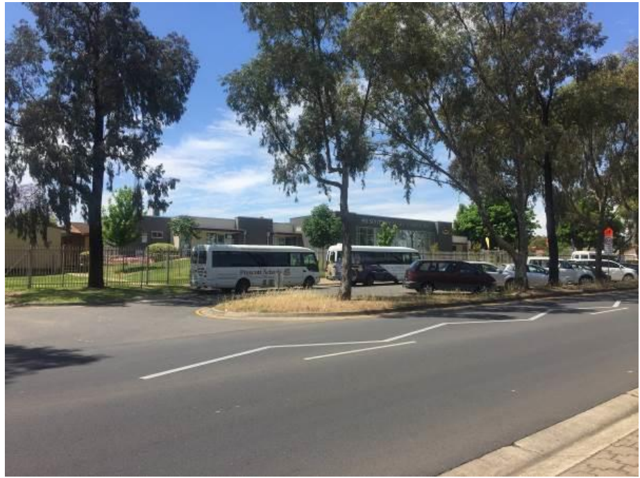
Photo 1. Looking north-east on Wright Road towards front of the school and car parking bays
