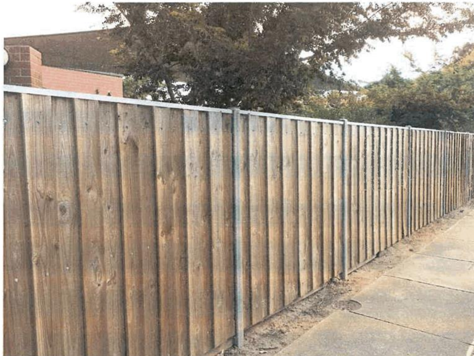
Image 1: Indicative boundary fencing along Evan Avenue.
