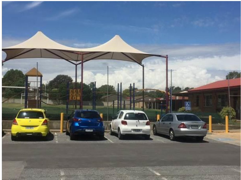
Photo 4. Looking east from the car park into the school grounds where the class room is to be constructed
