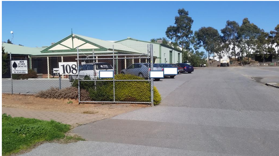
Photo 1. Looking south into the subject site towards the office and workshop
