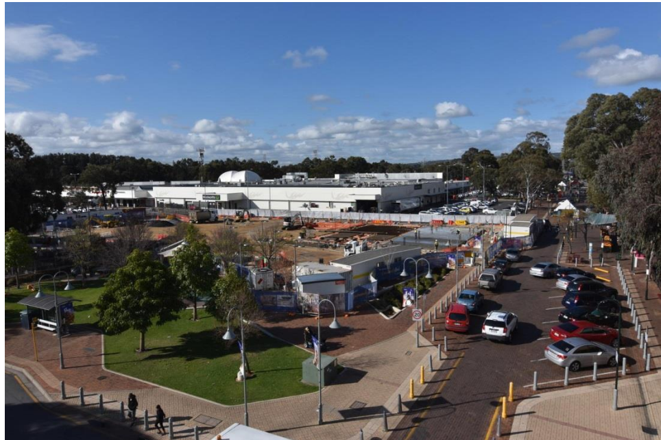
Photo 2: First concrete pour Ground Floor Slab (Photo: 19 September 2018)
