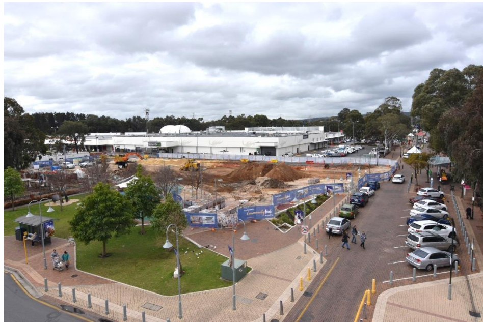
Photo 1: Civil earthworks commenced (Photo: 7 August 2018)
