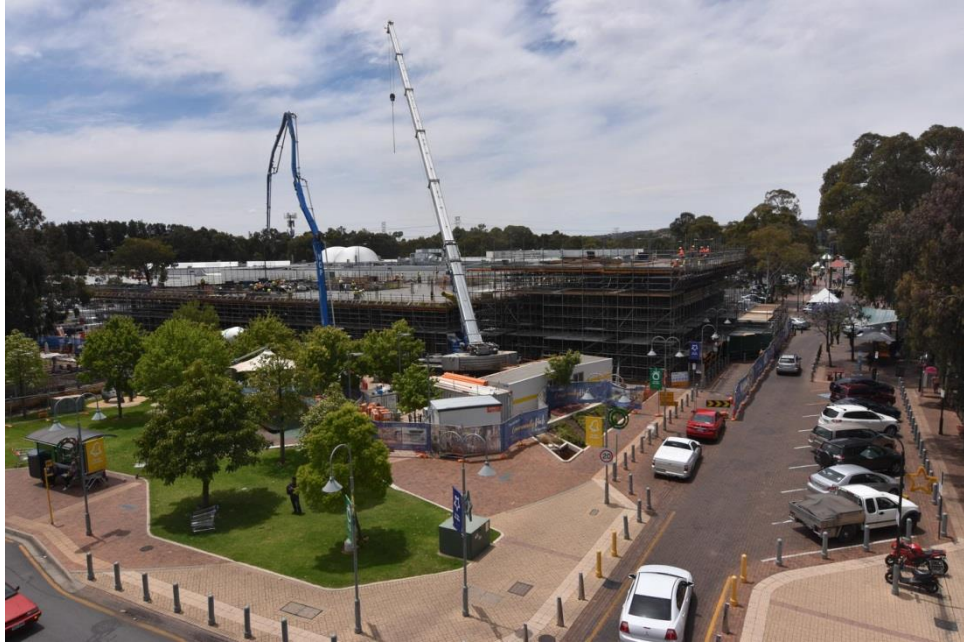
Photo 3: Level 1 second concrete pour; Level 2 Formwork (Photo: 27 November 2018)
