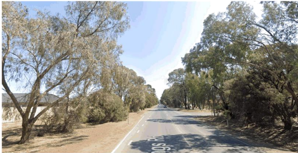
Photo 7: Looking west along Kings Road
