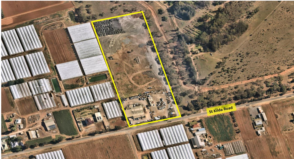
Panorama View – Looking South towards Subject Site (Source: NearMap)
