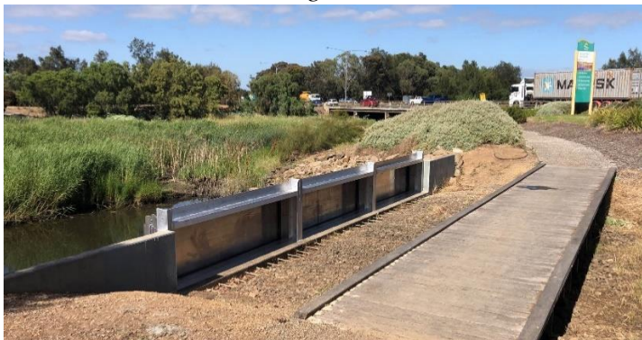
Mawson Lakes Flood Mitigation Works
