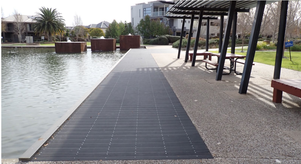
New decking at Bridge 186 Cascades, Mawson Lakes
