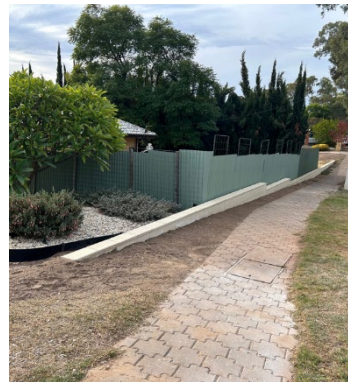
Retaining wall at 9 Wilson Road
