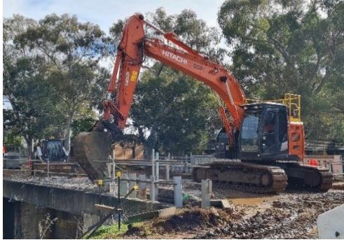
Pratt Avenue Bridge, Pooraka,
