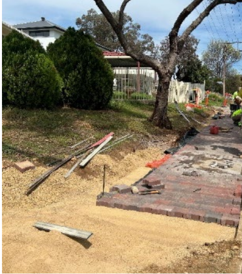
Fairfax Road, Ingle Farm, Footpath Upgrade
