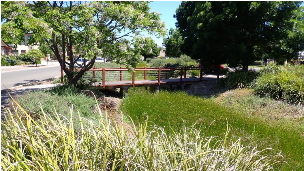
Example - Footbridge, BRIDGE-221 Hindmarsh Circuit Reserve, Shoalhaven Village, Mawson Lakes
