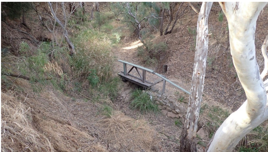
Example - Hiking Trail Bridge BRIDGE-204 Cobbler Creek Reserve, Salisbury East / Salisbury Heights
