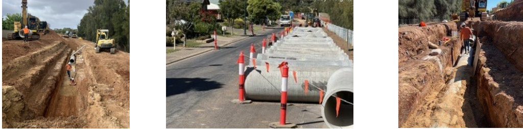
Brickwork Place, Walkley Heights, Flood Mitigation Works
