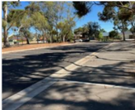
Parafield Gardens Oval Carpark Renewal
